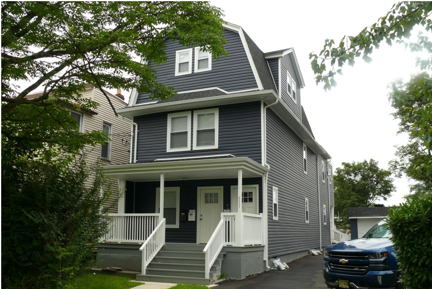
111 Maple Avenue: 1910, Colonial Revival, Contributing
